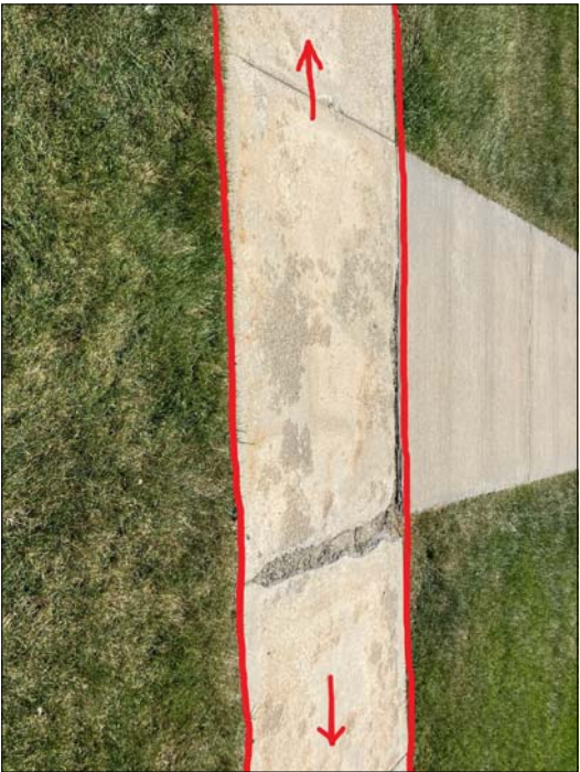
01 NORTH OF BLDGS. 3325 AND 3345 SIZE: APPROX 280 LINEAR FEET OF 4" SIDEWALK
